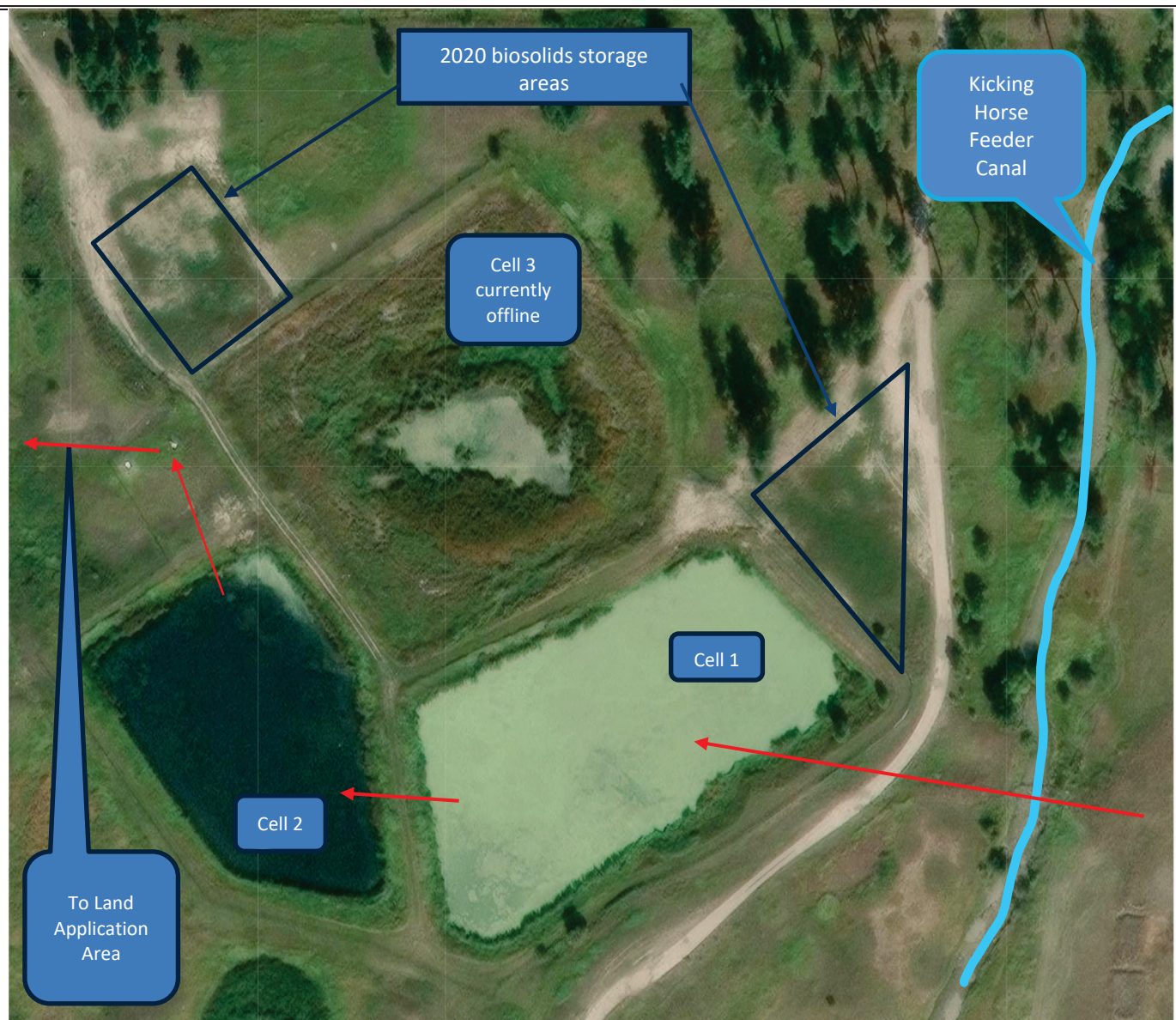
Kicking Horse Job Corps Wastewater Treatment Lagoons
