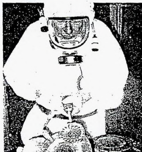
Fig. 4 (top): Removing an after service asbestos-containing gasket from a pipe flange by hand-scraping.
