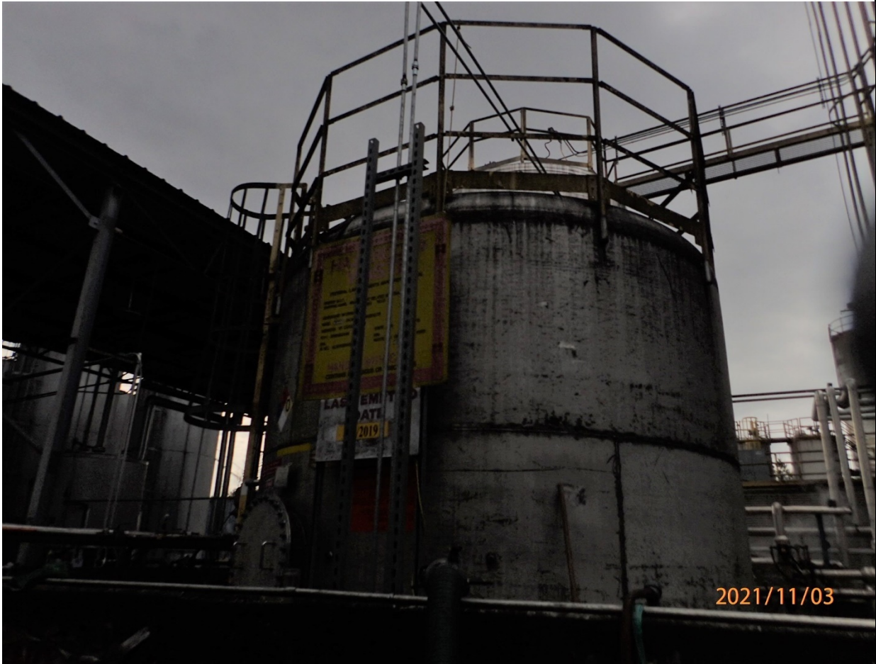
Photo 10: Tank 58 12,000-gallons, was labeled “Hazardous Waste” “Dirty Thinner” and marked with an indication of hazard.
