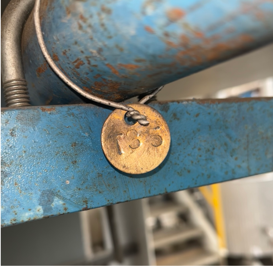
Photo 9: Illegible tags were cleaned, and photos of the tags were submitted to the inspectors on the day of the inspection.
