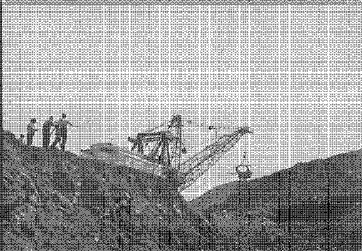
The big dragline in operation, with the engineers surveying a stripping bank.
