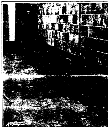
Lead shower pans installed in the new Chicago Post Office before receiving coats of asphaltum and shower floors.
