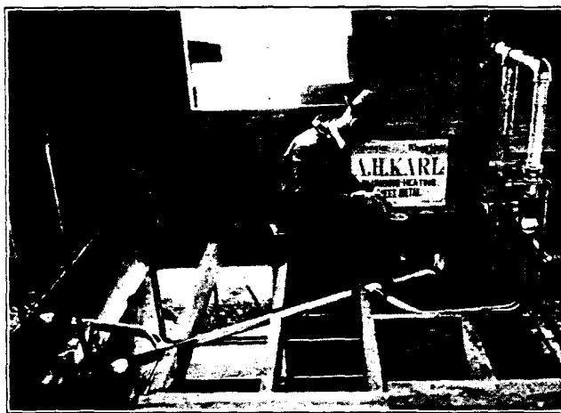
Lead wastes in a Mt. Vernon, N. Y., home. Screw pipe for the same installation would have required eighteen threaded connections as against six wiped joints in lead.
