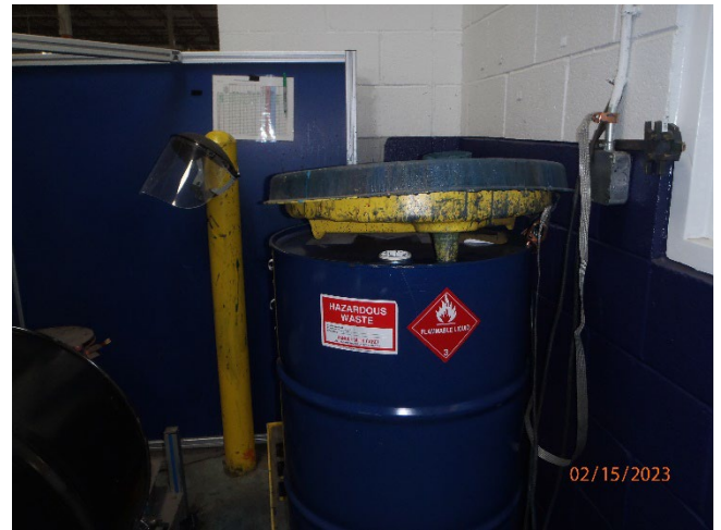
Figure 23: P2150037.JPG – Container of Acetone outside the Printing Room
