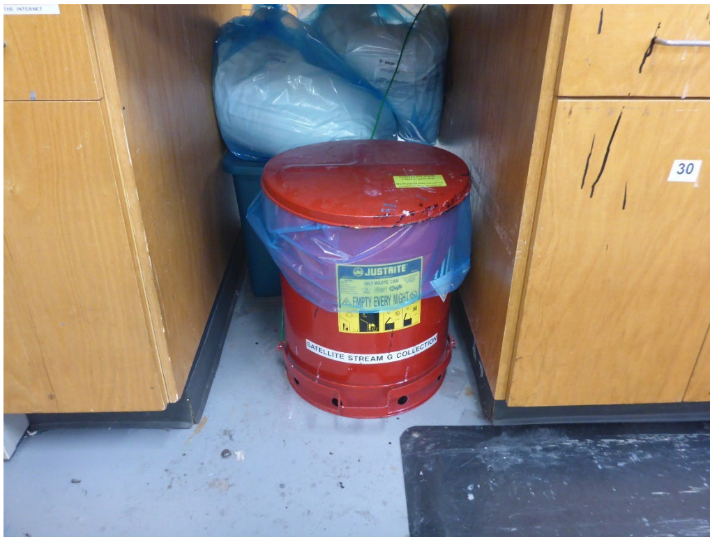
Photo 14: One of four 14-gallon step-to-open flammable cans in the Film Laboratory SAA for accumulating Stream G hazardous waste solids. The container was not labeled “hazardous waste” or marked with an indication of the hazards of its contents. In addition, the original “oily rags” and “empty every night” labels are still visible on the container.
