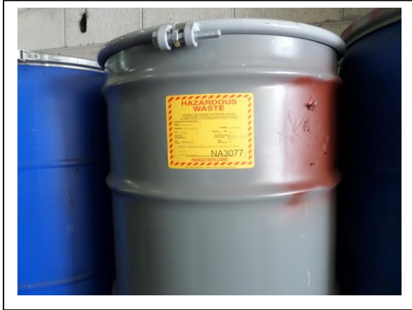
Metal Coaters. Universal Waste Accumulation Area. Inspectors observed a 55-gallon container accumulating hazardous waste crushed lamps with no hazard indicator. Photograph 17 taken at 12:01 p.m.
