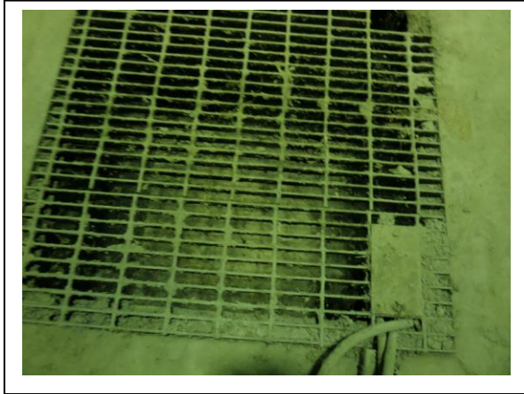
Metal Coaters. Solvent Storage Room. Inspectors observed floor level concrete sump. Photograph 21 taken at 12:09 p.m.
