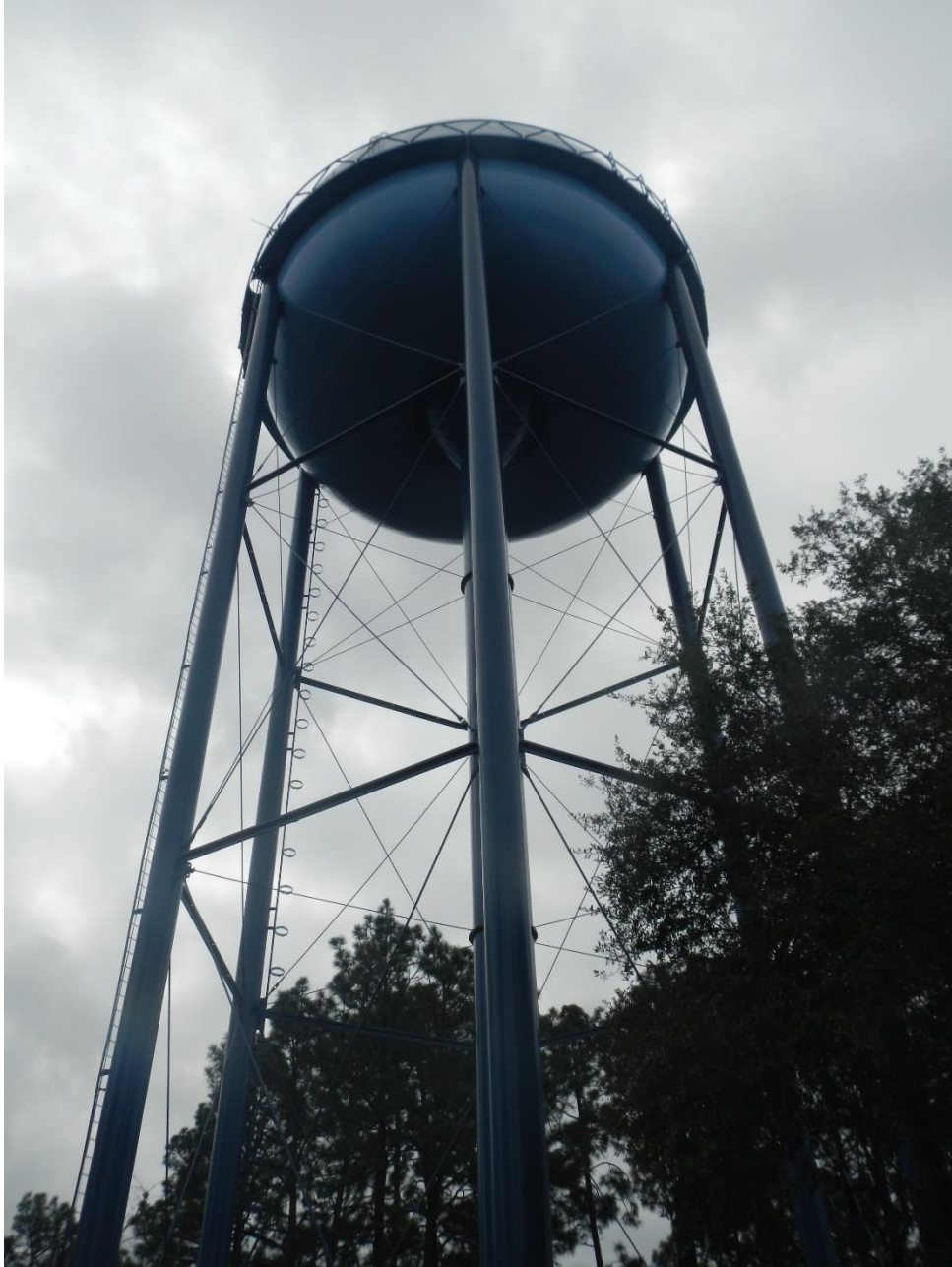
Photograph 5: Pony Hill elevated storage tank with vegetation in the vertical plane.
