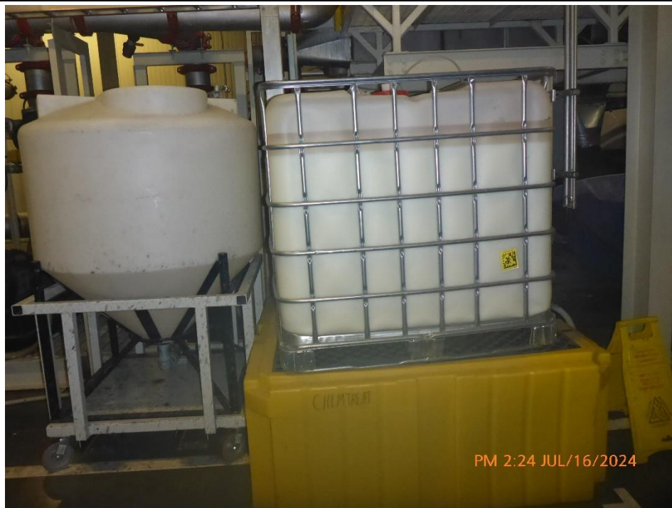
Photograph 5: Chemical tote in the paint shop observed to be partially on secondary containment.
