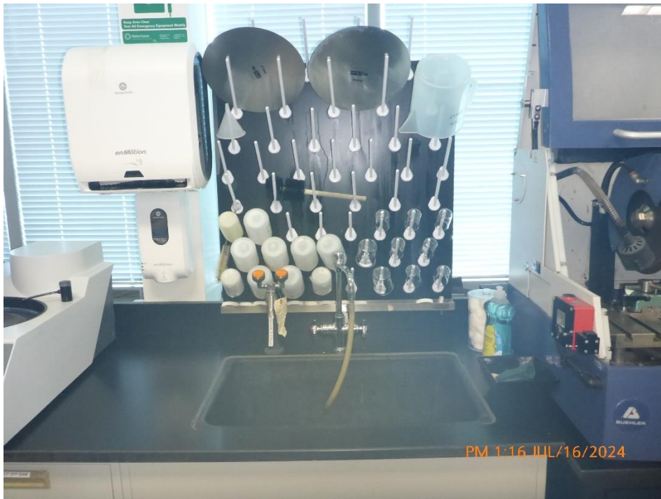
Photograph 4: Sink in the quality lab that discharges to the wastewater treatment process.
