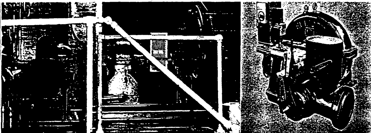
The drive for No. 2 paper machine is an Elliott 250-hp, single-stage turbine. Since this installation photograph does not show detail well enough, a shop view of this turbine, which is equipped with a special paper-machine-drive governor, is shown at the right.
