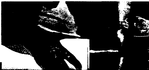
J-M PLASTIC COUPLINGS (left) make it easy to rapidly assemble successive lengths of Transite Ducts. They form a silt-tight joint and assure correct duct alignment. These couplings also permit slight changes in direction.
