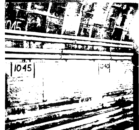
Transite Korduct safeguards many cables against fire
