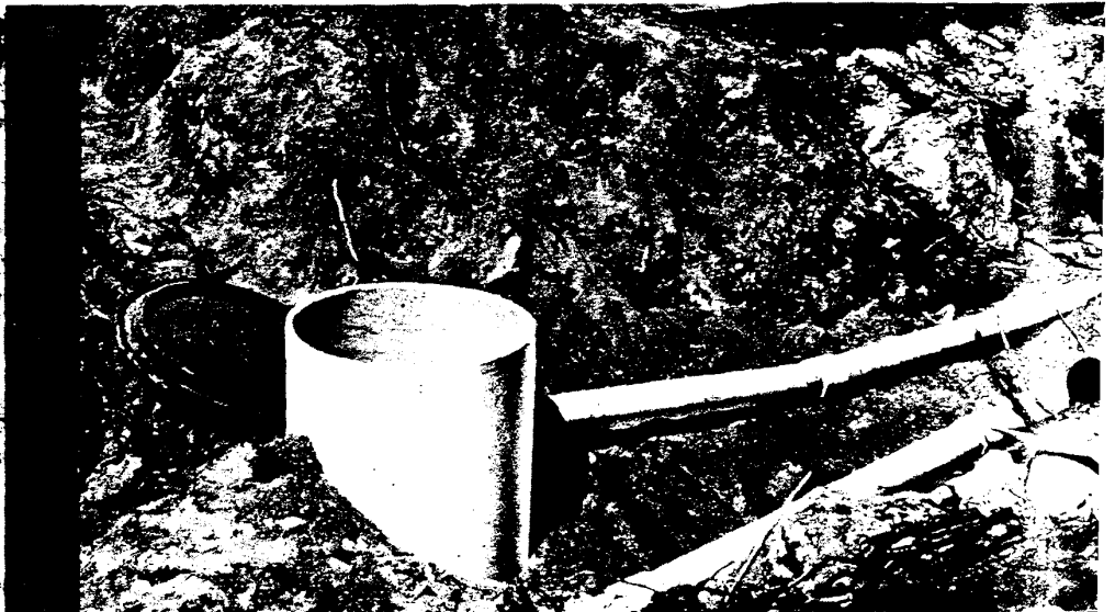
Transite Conduit and a Transite Pipe Service Box during installation in an Eastern Residential Community.
