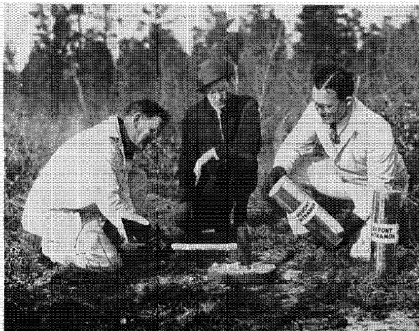
Demonstrating that "Nitramon" will not explode even when pounded repeatedly with a sledge hammer. Left to right, Charles Bennett, Dr. W. E. Kirst, assistant director, Eastern Laboratory, and Paul Sweeney
