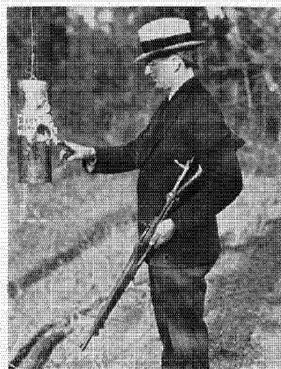
ACME The effect of shooting bullets into a can of "Nitramon" with an Army rifle. There was no explosion. D. M. Carr, of the du Pont Company was the marksman.
