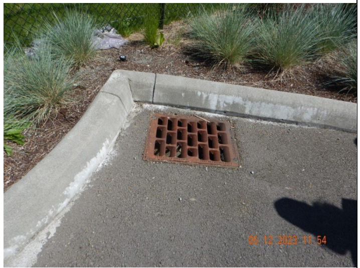
Photo #: 02 (DSCN0604) Description: Facing north, catch basin at perimeter of facility. Stormwater flows north into nearby retention basin.
