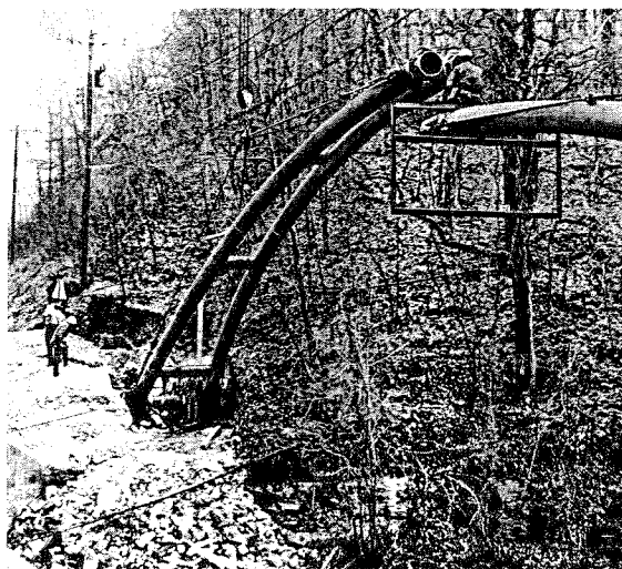
PIPING FABRICATION —This 150-foot self-supporting arch is part of the distribution system of Laclede Gas Company of St. Louis. Completely prefabricated in the shops of Midwest Piping, it was erected in one day. The installation is capable of carrying 200 million cubic feet of gas per day, at a pressure of 880 pounds per square inch.
