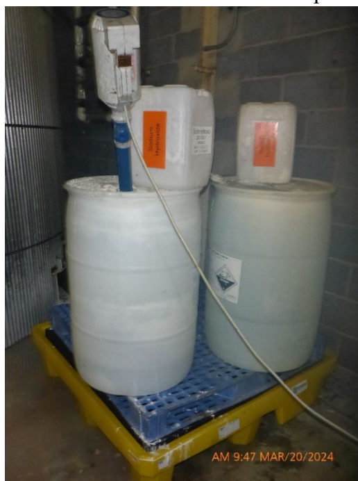
Photograph 5: Sodium hydroxide stored partially on secondary containment at Arxada.
