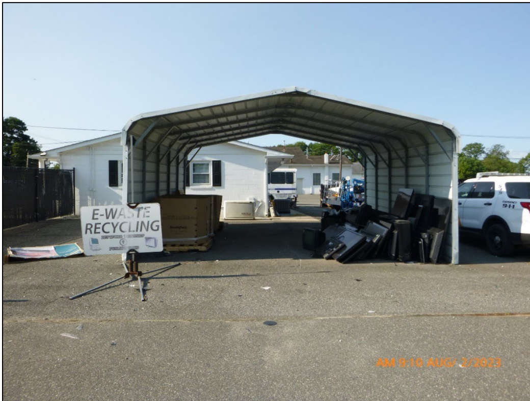
Photograph 12. Department of Public Works – View, facing south, of the structure that houses “e-waste recycling from residents”.
