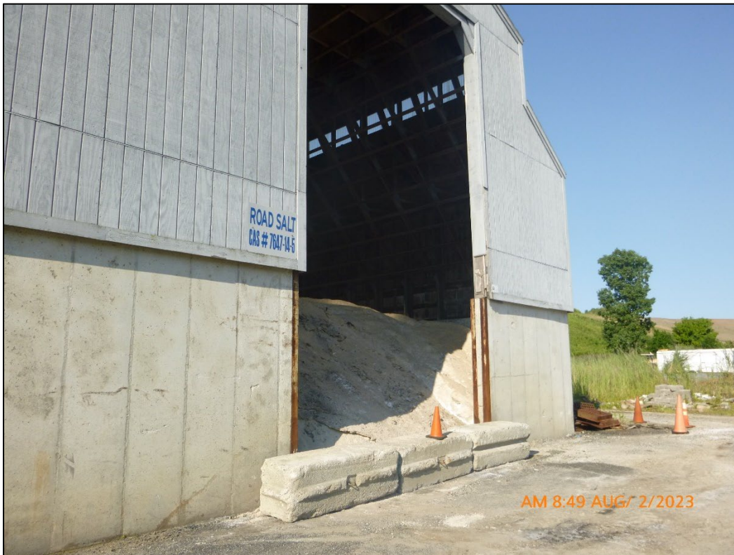
Photograph 4. Department of Public Works – View, facing southwest, of the salt shed.
