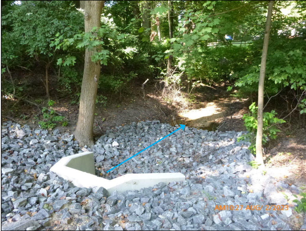
Photograph 15. Carson Avenue Stream Scouring – View, facing south, of the rip rap installed to mitigate stream scouring.
