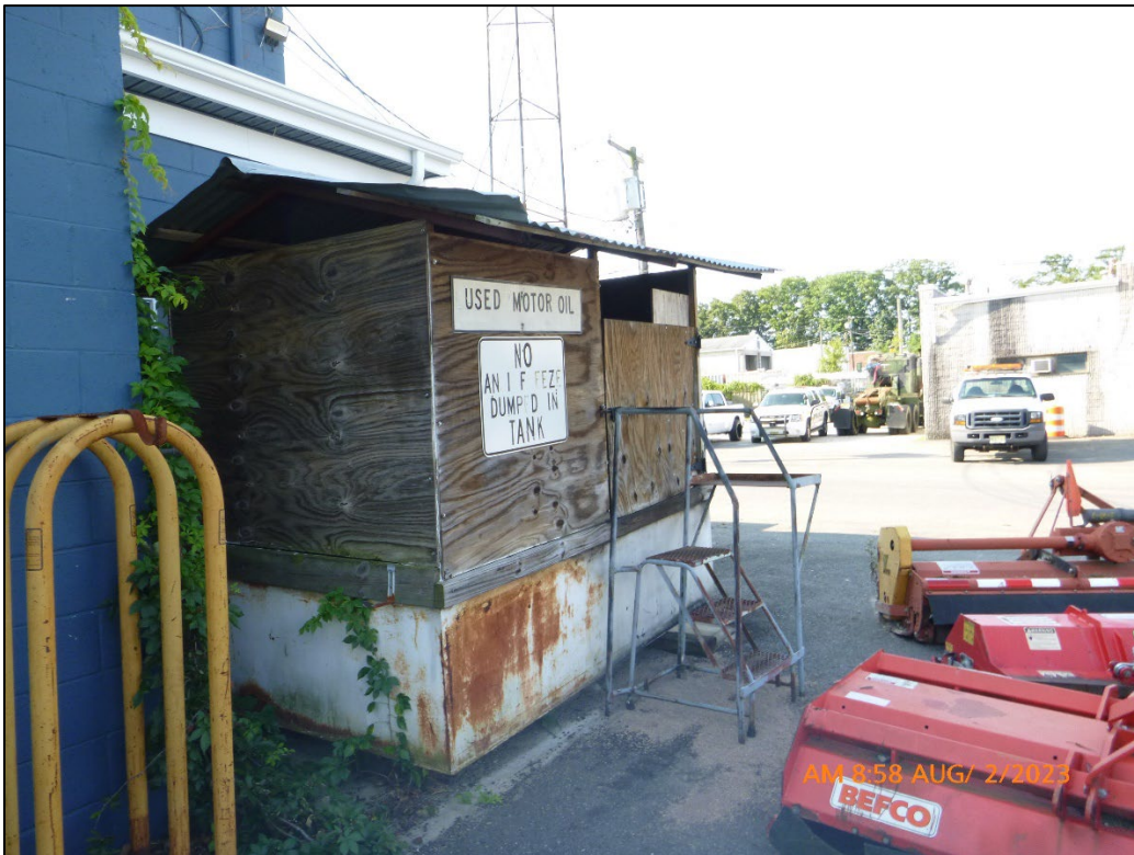
Photograph 10. Department of Public Works – View, facing southeast, of the structure housing the waste oil tank.
