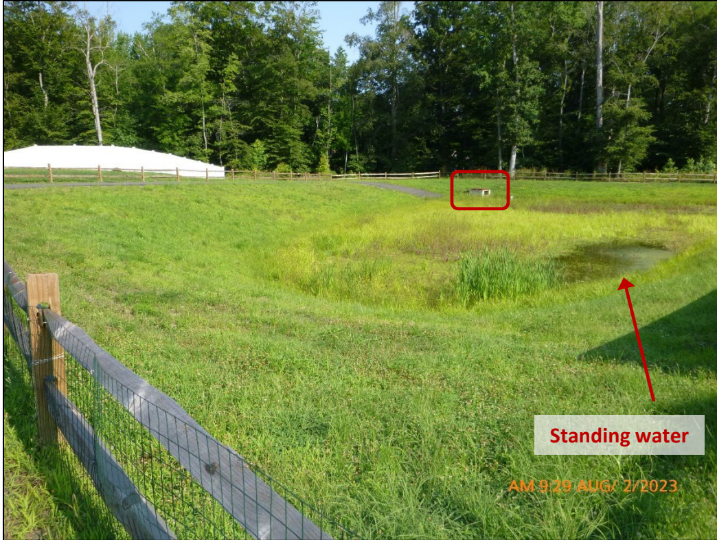
Photograph 13. Heritage Basin – View, facing north, of the detention basin. The weir structure is in the northern corner (red). Note the standing water.
