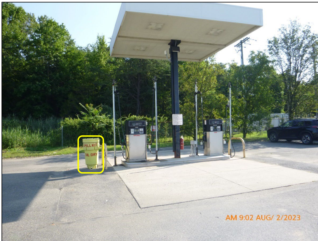
Photograph 6. Department of Public Works – View, facing north, of the fuel pumps and spill kit (yellow).
