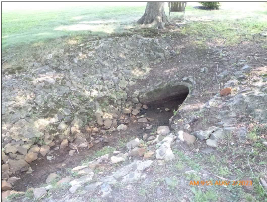
Photograph 14. Lake Bridge Community – View, facing southwest, of outfall B005.
