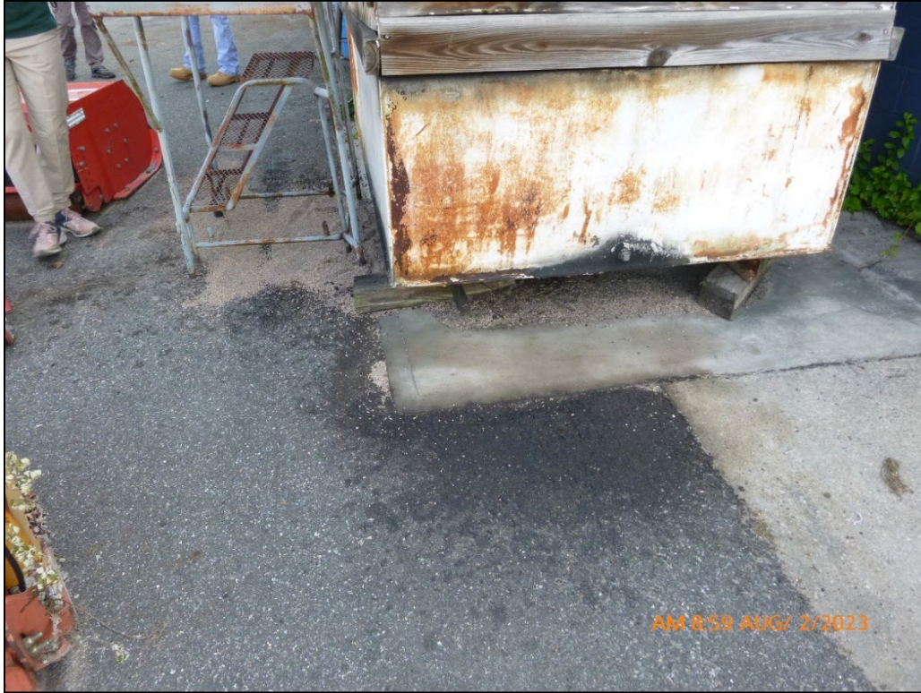
Photograph 11. Department of Public Works – View of the ground surface around the waste oil tank structure. Oil was observed spilled on the ground around the tank.
