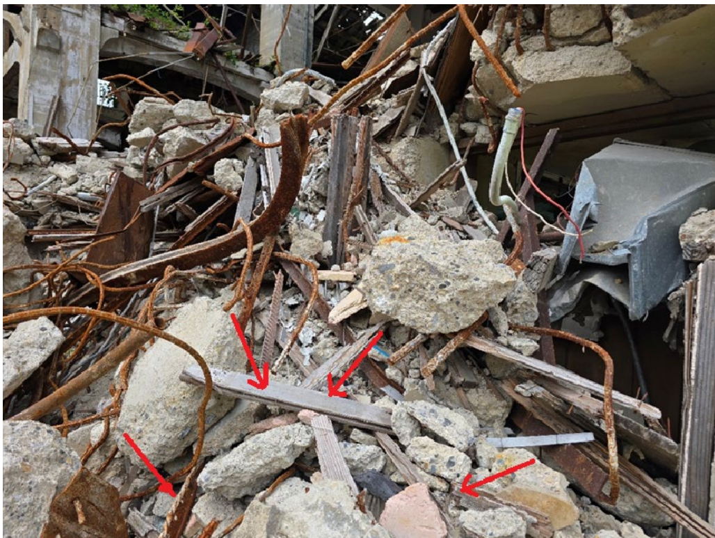
Figure 6: ACM laying in debris pile from Figure 4.
