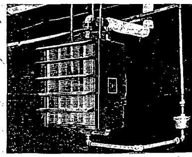
No. 30 Armstrong Trap keeping Unit Heater free of condensate and air
