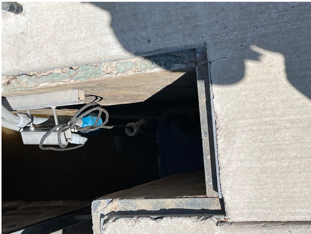
View inside the onsite lift station after the hatchway had been opened. (IMG_0371) Photographed by D. Esparza. 09/18/2025 (1:23 PM)
