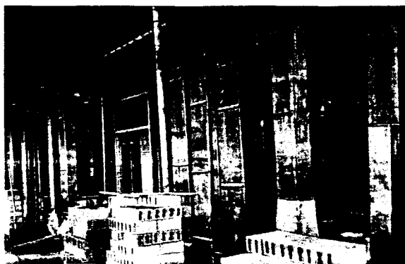
Some of the lead risers in the chemical laboratory ventilating system, giving an idea of the vast extent of the installation.
