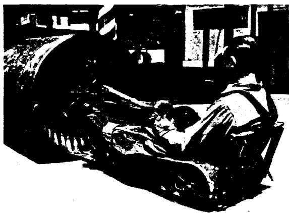
Two views of the storage-battery-operated car used to inspect pipe line enamel by Los Angeles Bureau of Water Works and Supply.
