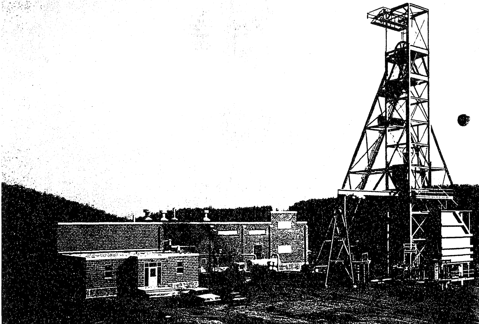
Shaft-sinking and development began during 1962 at No. 29 Mine near Viburnum, Mo. (shown above). When in operation, No. 29 will complete a trio of mines sending ore to Viburnum Mill, where capacity will be increased to more than 6,000 tons per day. Center of gravity of Missouri mining operations will gradually shift in the direction of new mining areas in and near Viburnum.
