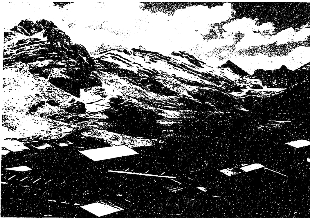
Spectacular surroundings characterize Santander Mine at 14,500 ft. in Peruvian Andes. Shown above are mill building with new rod mill in foreground, which has increased capacity to 700 tons of ore daily. Staff houses are at left, garage, shops and warehouse in center, lake for tailings in background.
