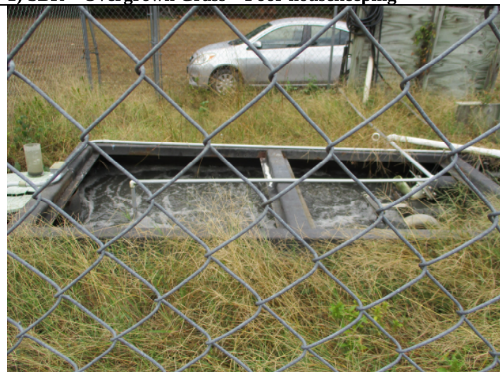
3) SBR Aerating and Overgrown Grass – Poor housekeeping
