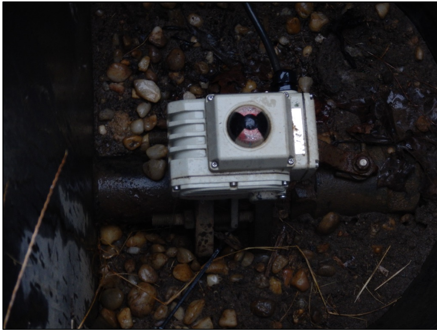
Photograph 7. Closeup view of the solenoid valve. Note that it was red, indicating it was closed at the time of the inspection.
