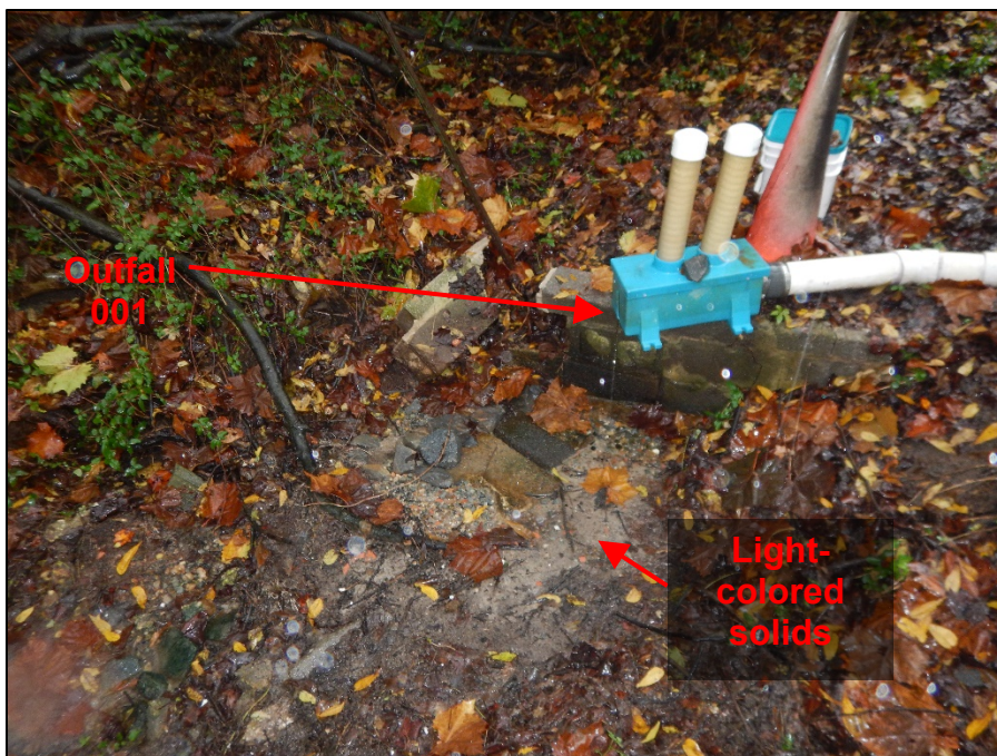
Photograph 12. View of dechlorination tablet feed at Outfall 001. Note the presence of light-colored brown solids just under the outfall.
