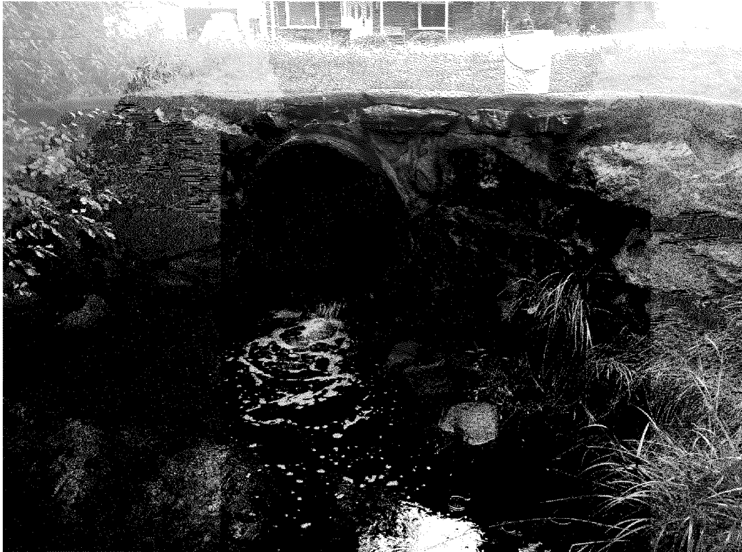
HasselBr: Outfall flowing south into Hassells Brook from under the street. Note the orange sediment on the bank in the lower right of the photo.
