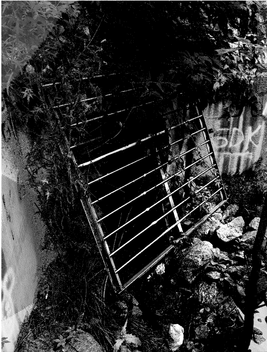
HarborAve: Outfall flowing west into Salmon Brook. Note the trash downstream of the outfall.
