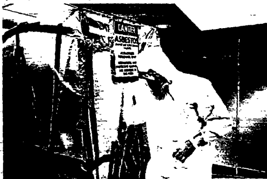
The risky, expensive process of asbestos removal is largely unregulated.
