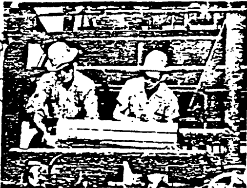
Insulators M. A. Gerald and J. W. Robertson of the Construction Department, in the picture at left, and the new aluminum-jacketed Thermobestos insulation system may be
