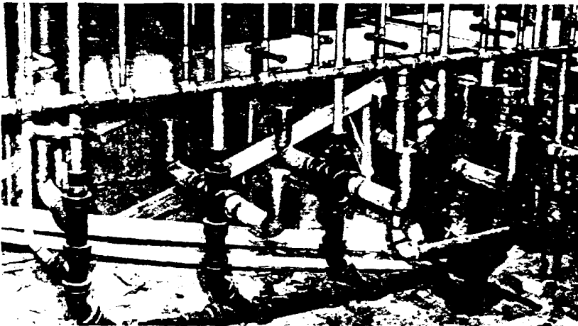
Lead bends and lavatory wastes in toilet room of American Airlines building in Tulsa, Oklahoma.
