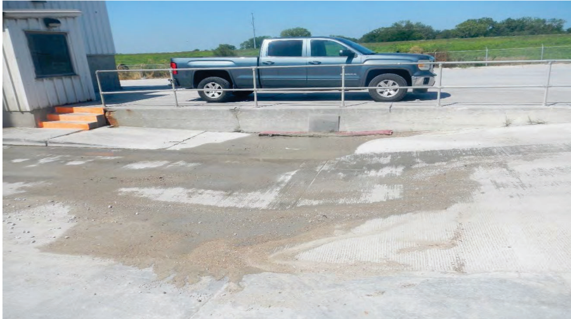
Photo 8, Inlet pipe connected to Outfall 02
