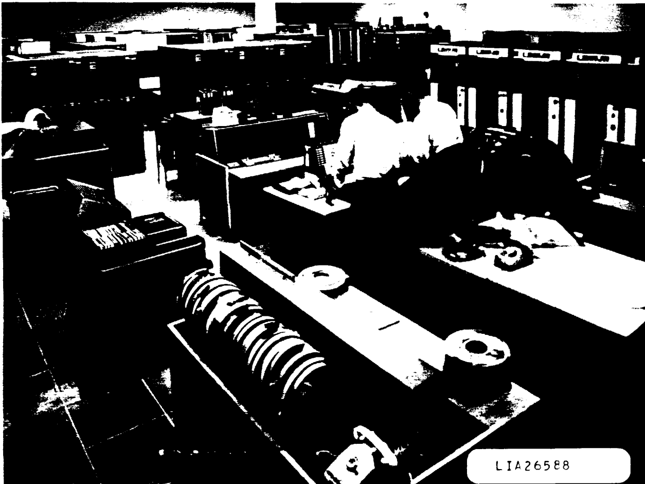
American's computer room showing its IBM 7090 Data Processing System. In the far background the IBM 1301 Disc Storage units are located.
