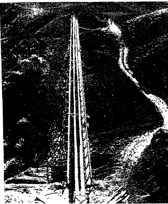
Belt conveyor line and tunnel from new sugar rock quarry
