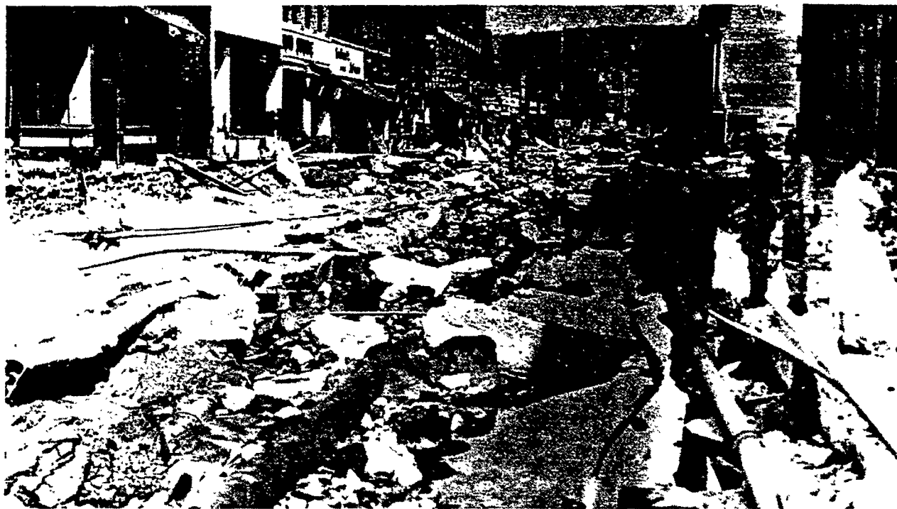
WATER MAIN withstood ravages of 1955 flood and continued in service at Winston, Conn.
