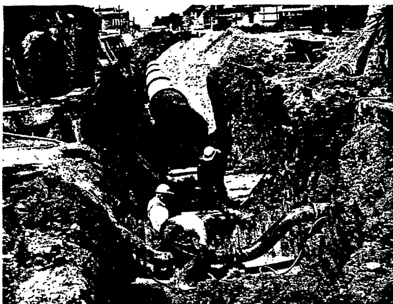
INSTALLING mains—42-in. roll-on-joint C.I. Pipe—Chicago, Ill. Placing offset in 8-in. main
