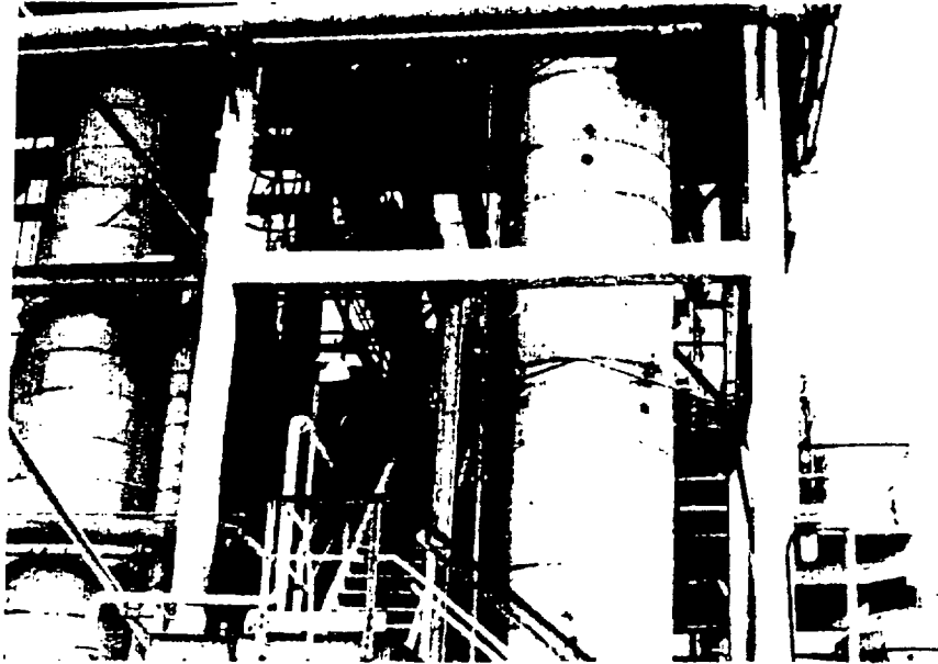
Figure 5. Structural fireproofing often contained asbestos materials.
