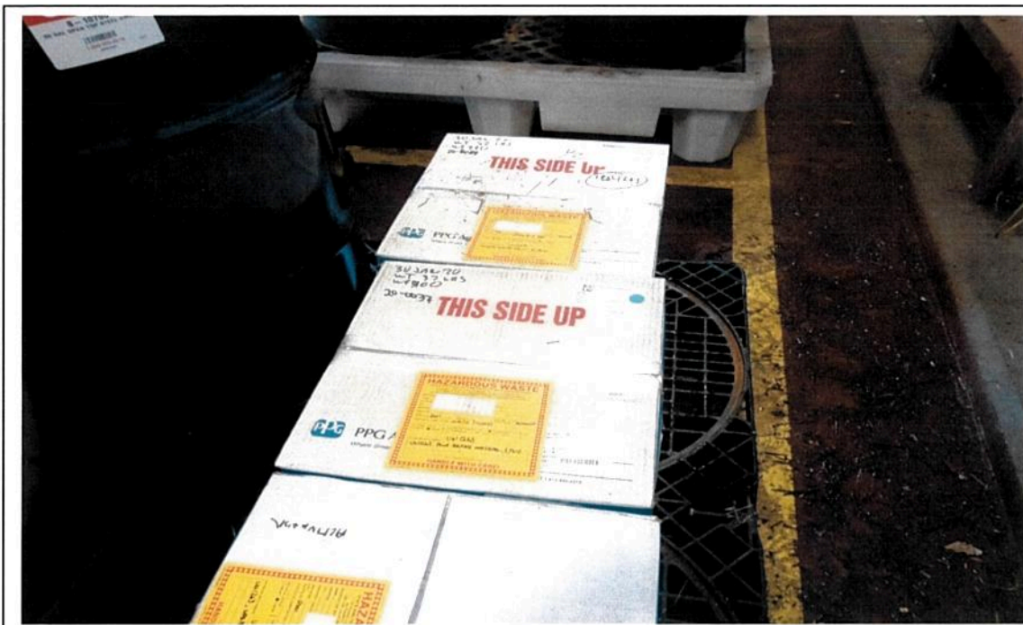
Naval Air Station Whiting Field. Main 90-Day or Less Accumulation Area Building 3156. Observed four boxes stacked two high on a poly pallet. Inspectors could not observe the hazardous waste label on each of the bottom boxes due to the double stacking. The facility removed the two top boxes revealing the labels. Photograph 2 taken at 10:16 a.m. WK.
