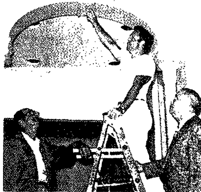
● FROM RIGHT are Arthur D. Hoppe, president of the firm; Wayne Beatty, plastering foreman; Jack Hasley, vice president and field superintendent; Wayne is showing how he joined an ornate piece of staff work to run mold—with perfect alignment
