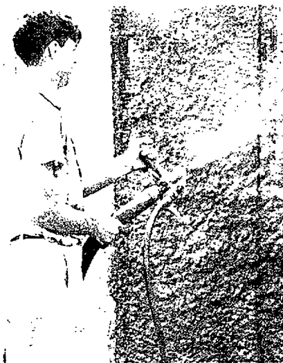
• NOZZLEMAN SCRATCHING metal lath with True Gun-All
