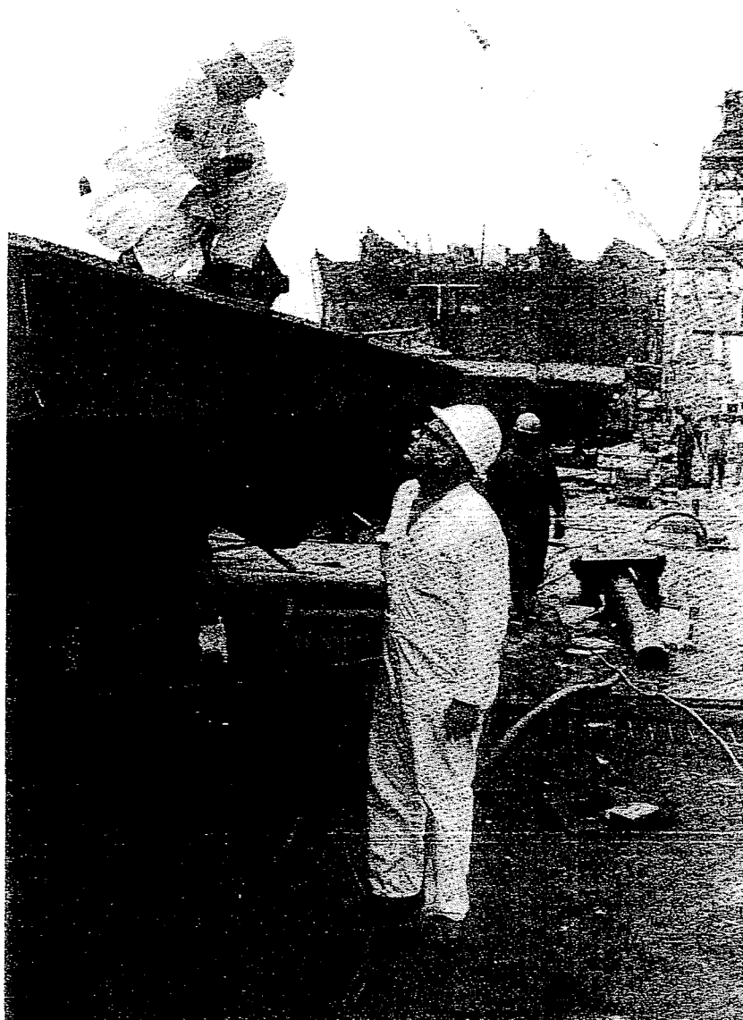
ESSO BATON ROUGE. Coating inspector Ed Worrel (top) and Bob Reed cross paths in sprawling Avondale shipyard where Esso Baton Rouge in background is beginning to take the shape of a ship under the watchful eyes of marine inspectors.
