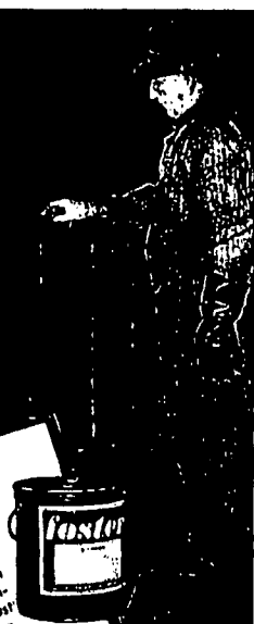
Application of H. I. Mastic to interior of boiler room (Foster Specification 1).
