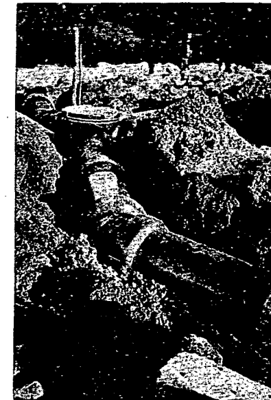
Large diameter clay pipe heating duct and plenum connection used in commercial structure. This type of duct, when installed in garages and maintenance or repair shops, can be used for heating, ventilating, air conditioning, and removal of exhaust gases. When the registers are located under the windows, the warm air will blanket the glass area and eliminate frosted and wet windows, sills, and walls.
