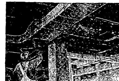
For Ducts. Light-weight blocks of FOAMGLAS were easily applied to these metal air conditioning ducts at the Moses H. Cone Memorial Hospital, Greensboro, North Carolina.
