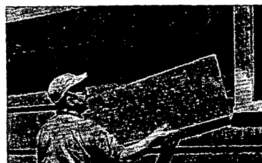
Applying shingles and Shingle-Backer
