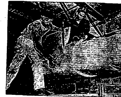
Microlite and Super-Fine can be fitted quickly around the duct and supporting hangers. Light-pauge wire ties complete the job. Men like to work with L.O.F. Glass Fibers' insulation because it is so soft and flexible—so pleasant to handle.
