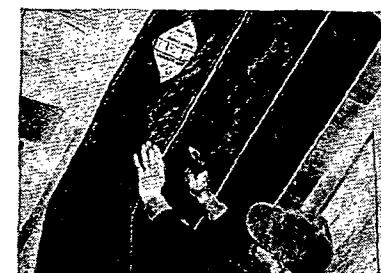
Applying Balsam-Wool Sealed Insulation
