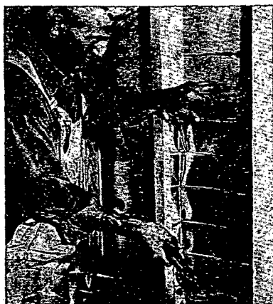
Ferro-Therm is Stapled Permanently in Place
