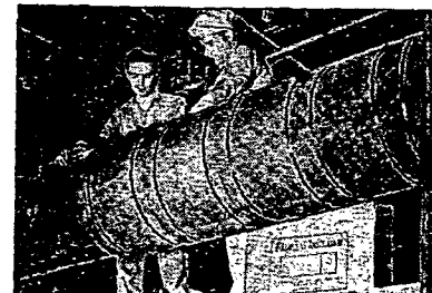
For Piping. FOAMGLAS pipe insulation (available for up to 36 in. pipe size) was applied on this welded pipe carrying cold water for the system air conditioning Pittsburgh's new Gateway Center skyscrapers.
