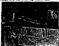
Positive seal of exposed sub-floor ends. Eliminates cold drafts and heat losses.
