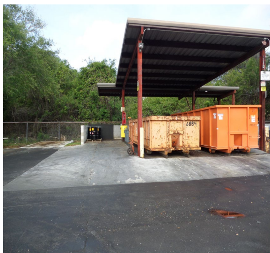
H & S Swansons Tool Company (H & S). 90-Day or Less Accumulation Area. Observed six 55-gallon containers accumulating hazardous waste. Photograph 1 taken at 9:47 a.m.
