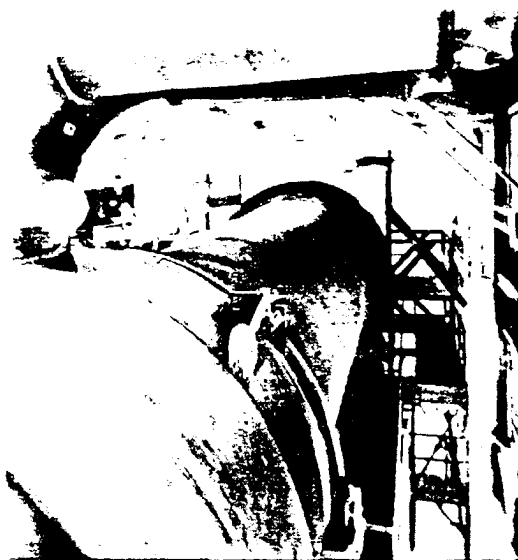
Rotary kilns where heat is applied to the processing of "Titanium" pigment.
