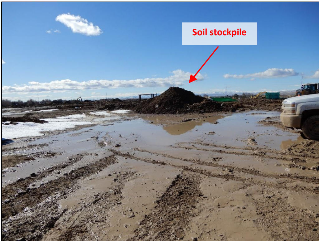
Photograph 2. View, facing south, of an unstabilized stockpile of soil located at the center of the Site.
