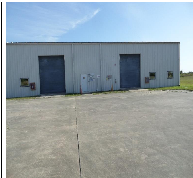
Cape Canaveral Space Force Station (CCSFS). Permitted Storage Building 44200. The inspectors observed signs posted on the building. Photograph 1 taken at 10:14 a.m.
