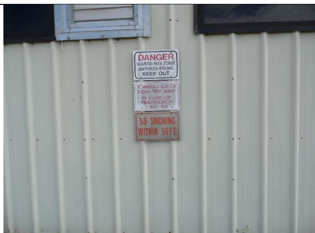
CCSFS. Permitted Storage Building 44200. The inspectors observed signs posted on side of the building. Photograph 6 taken at 10:55 a.m.
