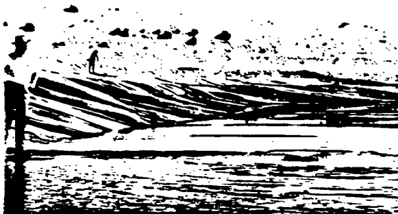
After outer edges of the lining are anchored in a trench, ponds are filled with water and are ready for use.
