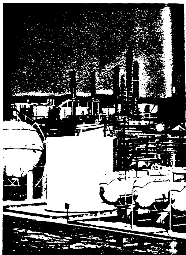
Vinyl chloride produced in these facilities at Ethyl's Baton Rouge plant—and at the Houston plant—is the chemical intermediate from which PVC is made.
