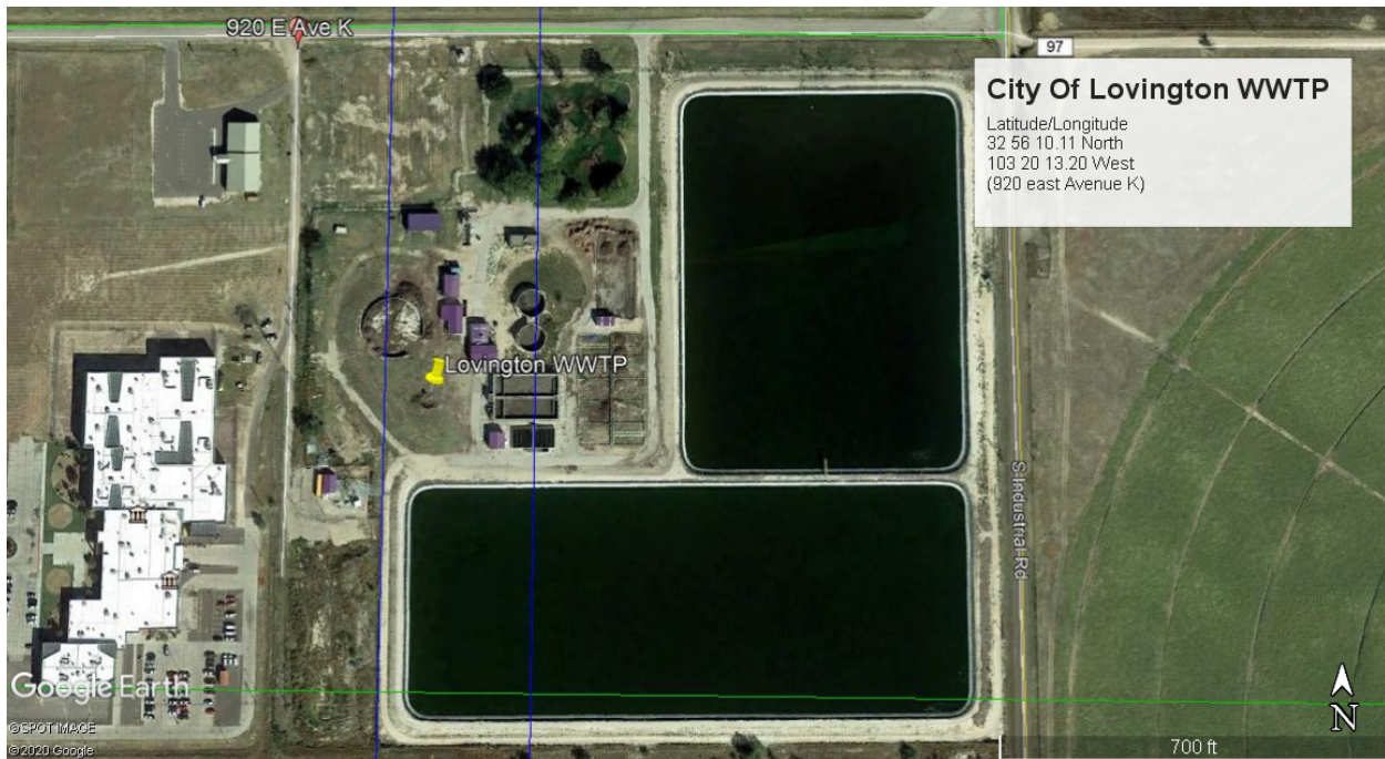
Aerial Image #1: Overall view of the City of Lovington’s Wastewater Treatment Plant and the two (2) disinfected effluent storage lagoons. Aerial from Google Earth maps.
