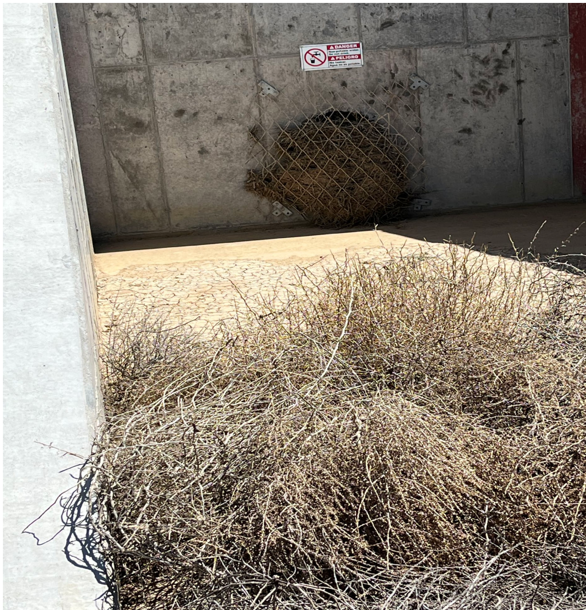
View of the CTPL discharge conduit. Note: It was recommended the vagrant debris be removed. (IMG_0056) (July 10, 2024: 2:57 PM) Photographed by D. Esparza
