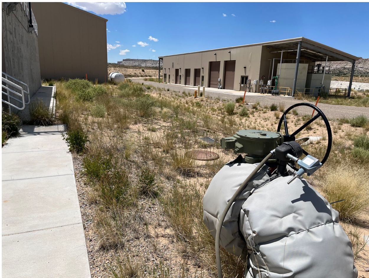
View of the location for future expansion adjacent to the existing flocculation/sedimentation basins. Looking approximately West. (IMG_0023) (July 10, 2024: 2:04 PM) Photographed by D. Esparza
