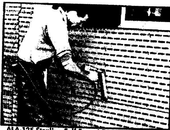
ALA-125 Stapling Self-Furred Exterior Stucco-Lath
