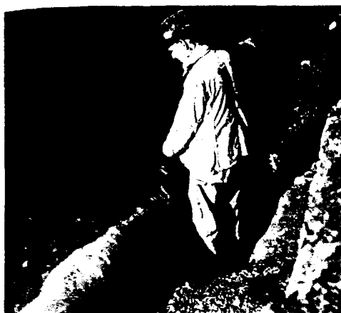
At left, calking part of the 20-in. cast-iron main for Chattanooga, and, at right, water department inspector examining lead-calked lengths of pipe
