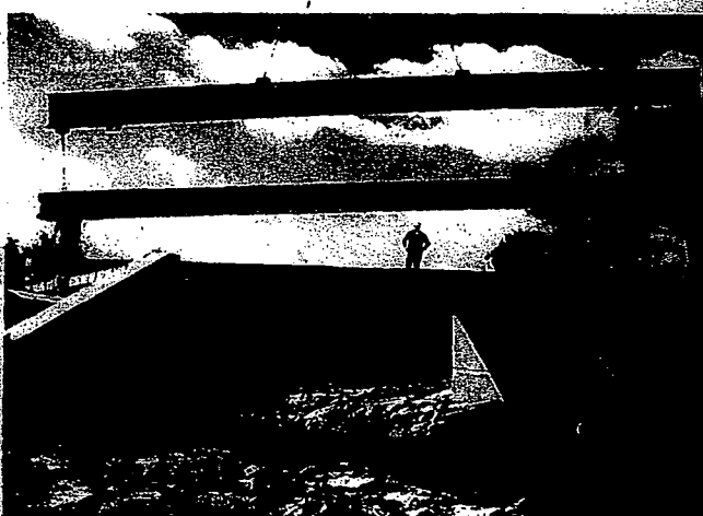
Precast replacement members lowered into place speed rebuilding.
