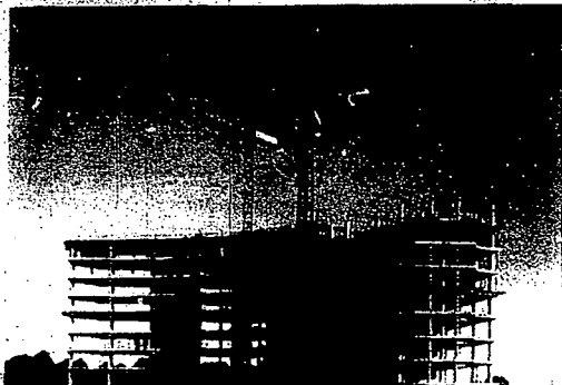
WK-226-SL Maximum capacity — 26,500 lb. Maximum reach — 196 ft Maximum freestanding height — 226 ft
