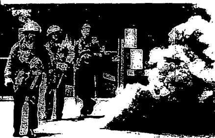
Smoke from transformer contained toxics.
