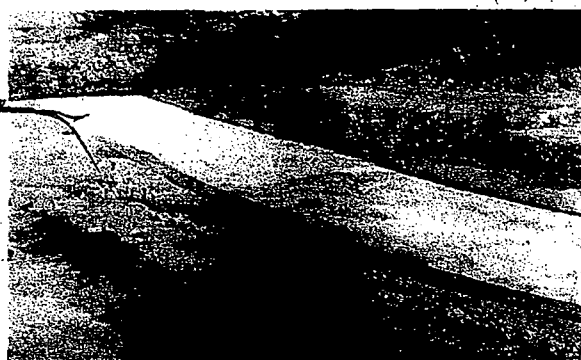
Plastic sheeting used to protect core during daily monsoon rains.
