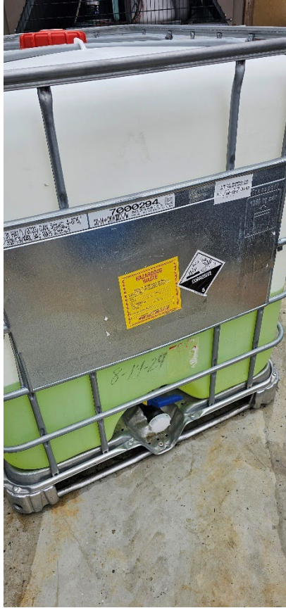
Figure 14: One 275-gallon hazardous waste tote located in the back pad area used to collect corrosive scrubber wastes was not dated. A date was observed written on tote for 08/14/2024 however, the facility representative stated the tote has been accumulating waste on site for approximately 6-months
