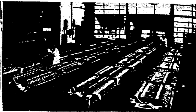
View of electrolytic cell room.
