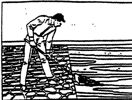
Sketch 13. Stand on the remaining floor covering, not the felt, during felt removal.
